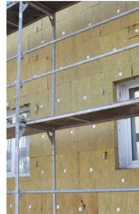
Image above credit: Decarbonising Camden's Existing Buildings A technical evidence base for planning policy for Camden Council by Etude, Currie and Brown. Image left credit: Katherine Frost – EWI being installed
